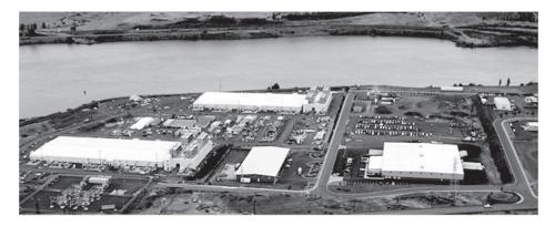
Figure 2.1 Photograph of Google's top-secret Dalles, OR data center, built near the Dalles Dam for access to cheap power. Note the large cooling towers on the end of each football-sized building on the left. These towers cool through evaporation rather than using more power-hungry chillers. Source: Melanie Conner, *New York Times*.
